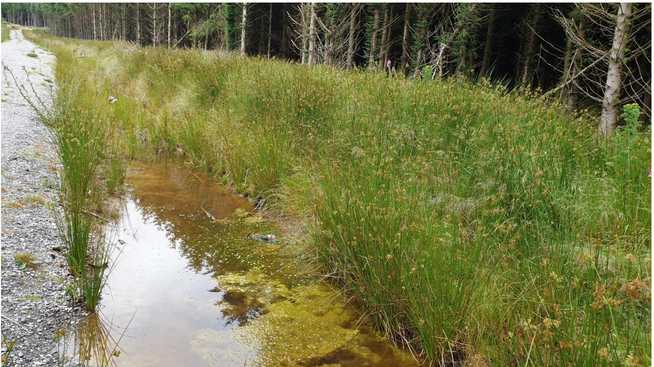
Plate 9.3: Example of Poor Drainage and Ponding at the Existing Roadside Forestry Drainage Near the T5 Hardstand Area of the Site
