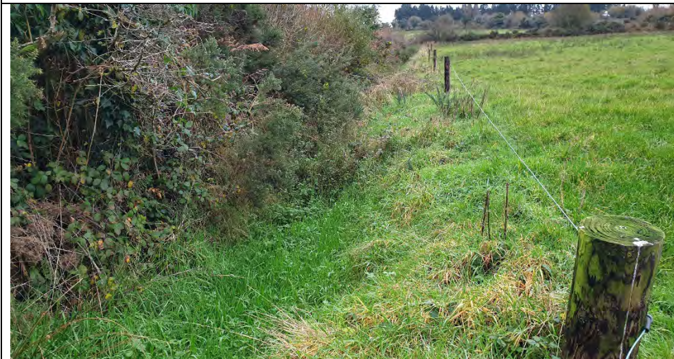
Typical Field Boundary Drain at the Central Area of the Site
