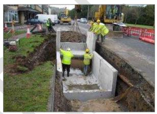
Figure 8 – Example of Joint Bay under construction (pre-cast)
