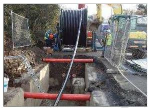
Figure 9 - HV cable pulling procedure (Drum set-up example)
