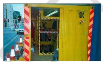
Figure 10 - HV cable jointing container
