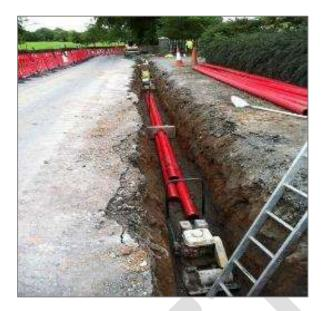
Figure 2 - Example of 110kV Underground Duct Installation
