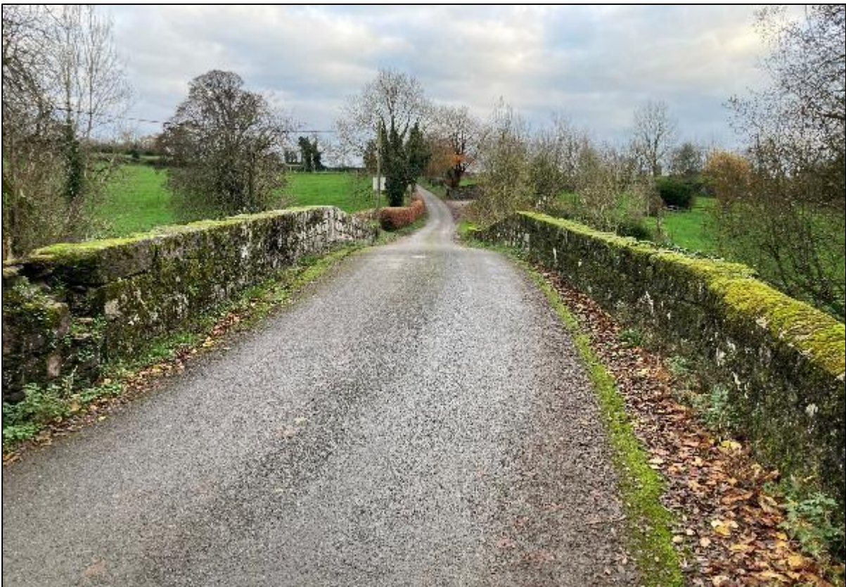
Plate 13.24 View of Mountain Stage Bridge (RPS ref. WA750688) from north
