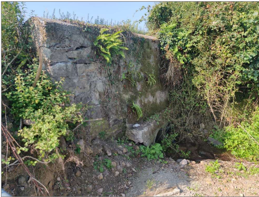
Figure 4 – Bridge A2 from the Northern side of the bridge
