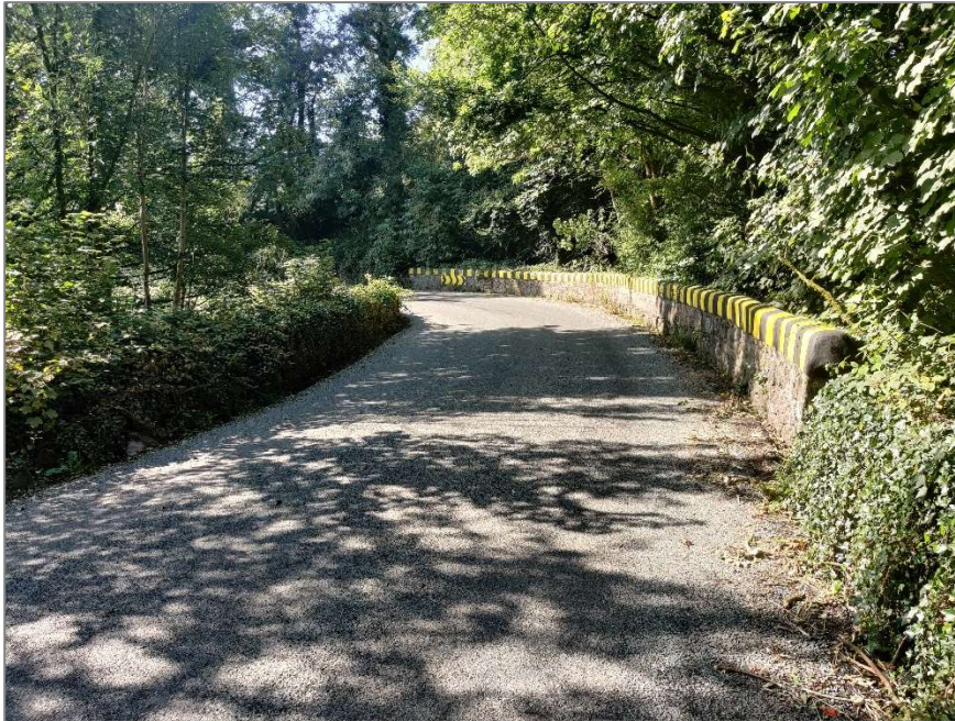
Figure 7 - Bride A6 View from North side of Bridge
