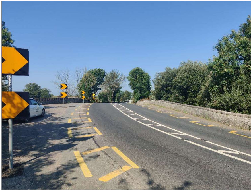
Figure 5 – Bridge A3 from the southeast of the Bridge
